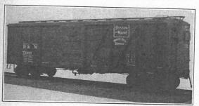
Equipment on these cars includes: Miner, Waugh, Durable and Durvea draft gears; National type "D" couplers; Buckeye Coupler Yokes; Ajax hand brake; Creco No. 2 plus brake beams; cast steel truck side frames with integral journal boxes made by
